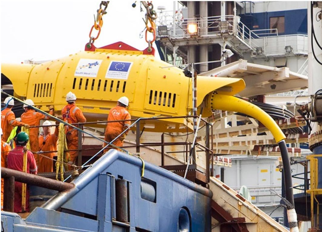
**Wave Hub unit being deployed 16km offshore from Hayle, Cornwall. The Wave Hub test facility is the world's largest and most technologically advanced site for the development of offshore renewable energy technology.**
