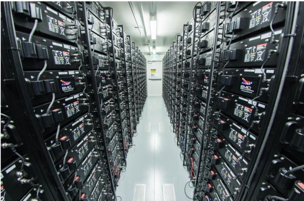
On-grid battery energy storage system (BESS) designed and delivered by Carnegie's Energy Made Clean subsidiary for the Western Australian State Government owned energy utility, Synergy.
